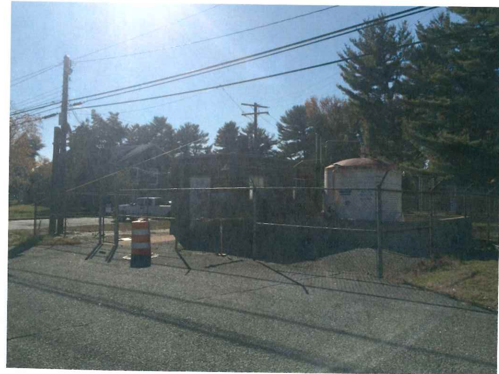
Photo 24: Former treatment building and treatment tank (currently out of service) along North Repauno Avenue on the eastern side of the property.
