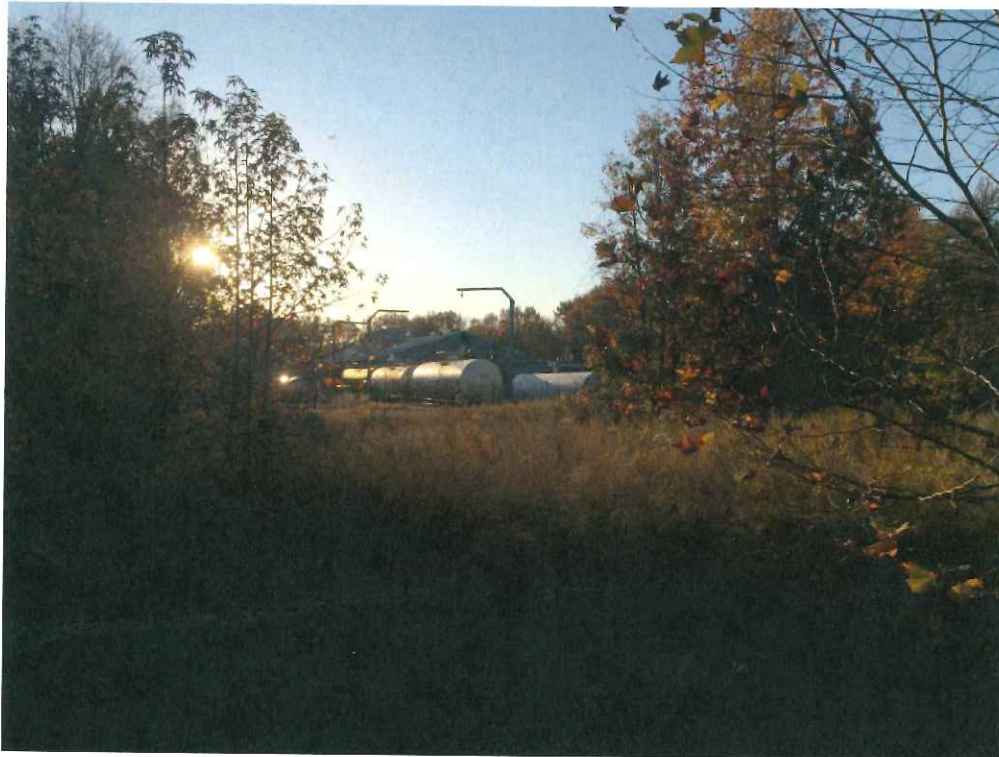
Photo 32: ASTs and rail cars at north adjacent ice plant.
