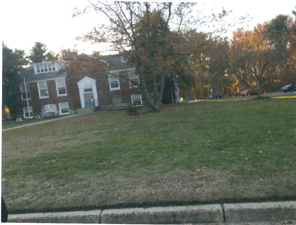
Photo 35: East adjacent property: Repauno Daycare Center
