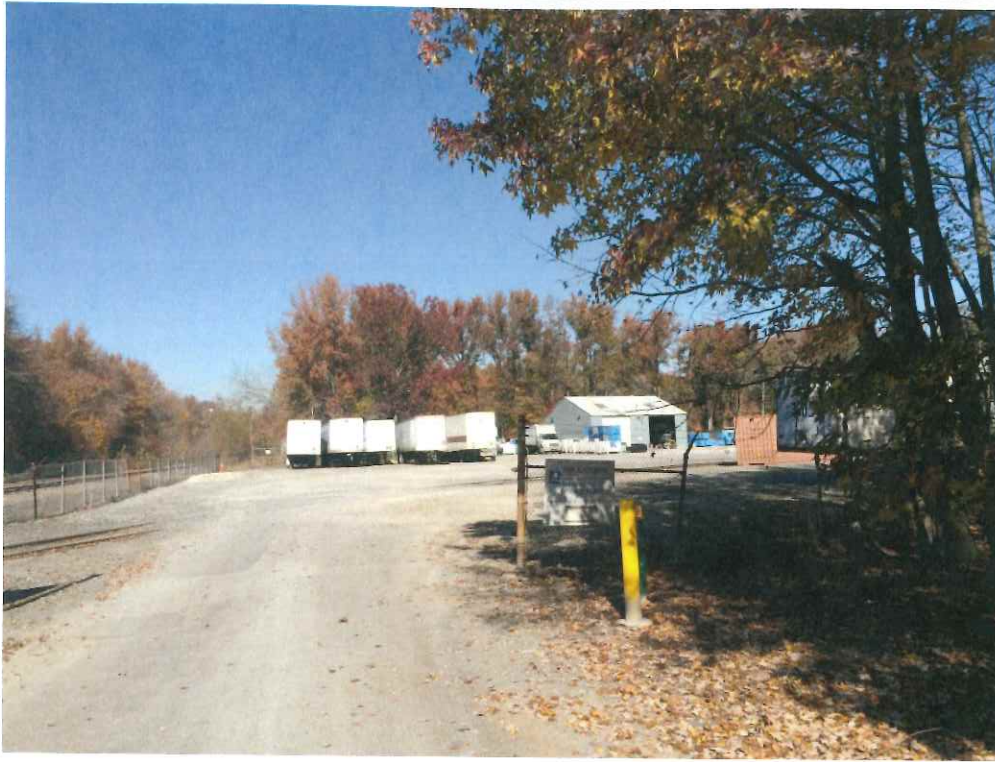
Photo 31: North adjacent ice plant.
